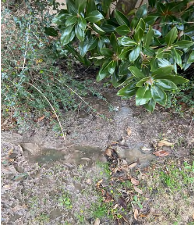
1. We received a call about sewer in yard.
