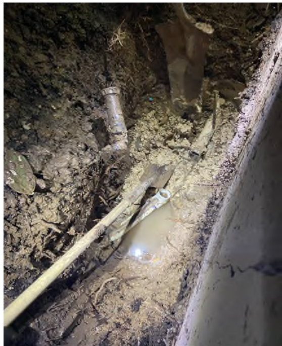
4. Removed exposed roots and damaged pipe.
