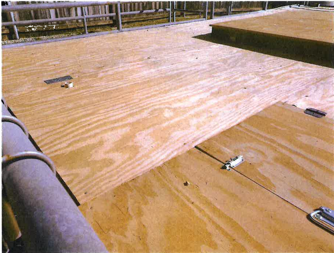
Figure 5: Plywood Decking - Minimal Fasteners in Place
