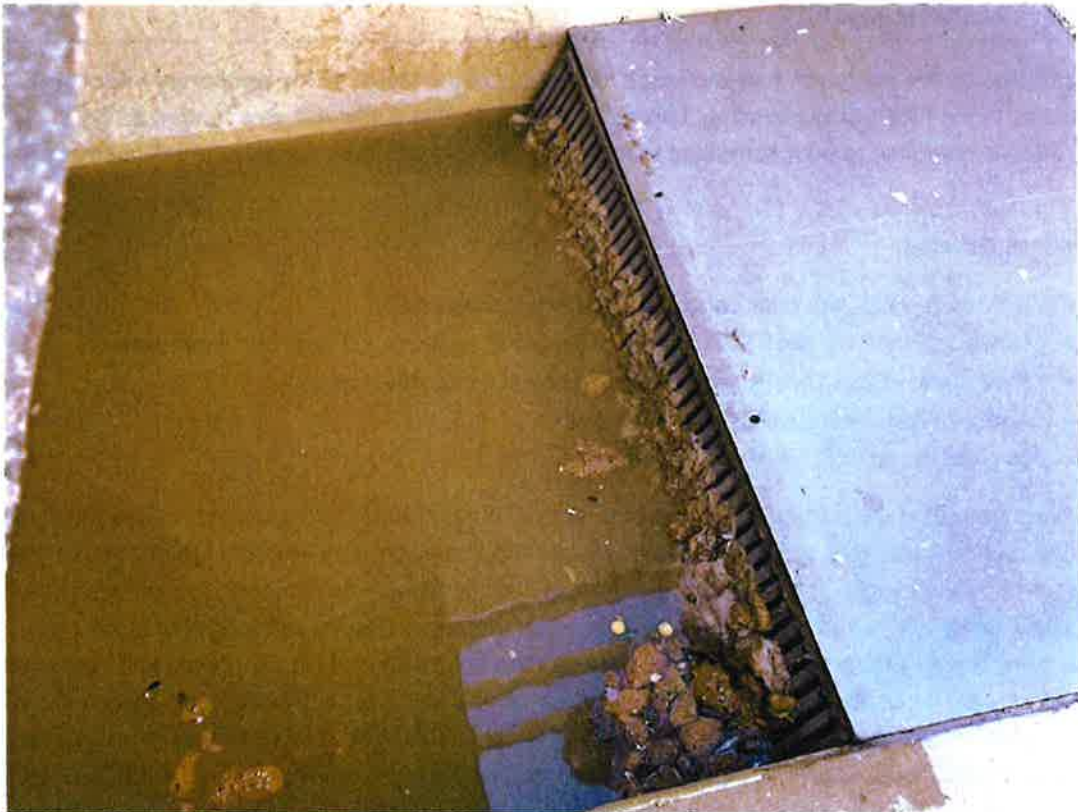
Figure 1: Significant (>90%) Blinding of Screen
