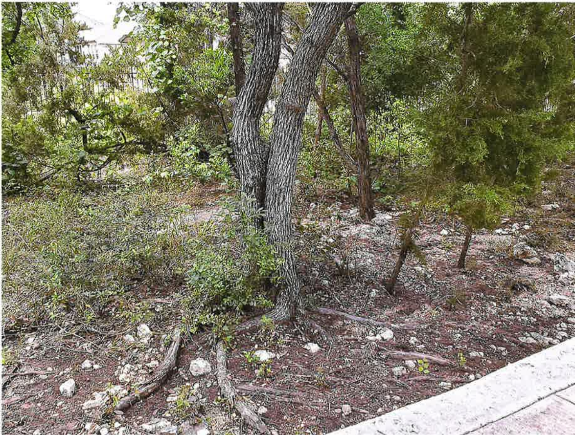
Figure 2: Example Erosion Caused by Overland Flow of Pond Effluent
