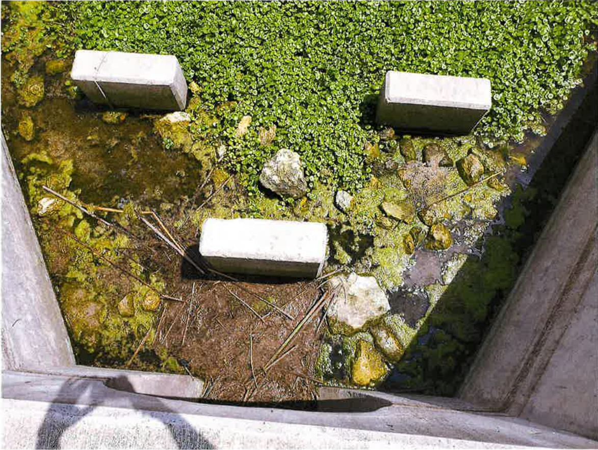
Figure 4: Rip Rap, Sediment, and Vegetation at Pond Inlet
