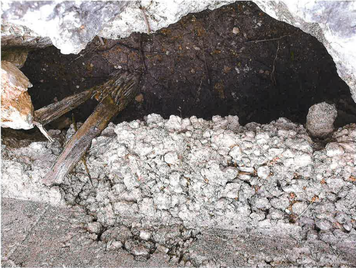
Figure 3: Example of Erosion at Outlet Weir
