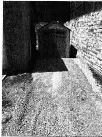
Polymer pump building
