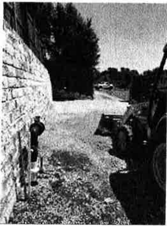
Sludge Box Pad site prep.
