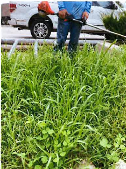
Drainage channel on Denise Cove
